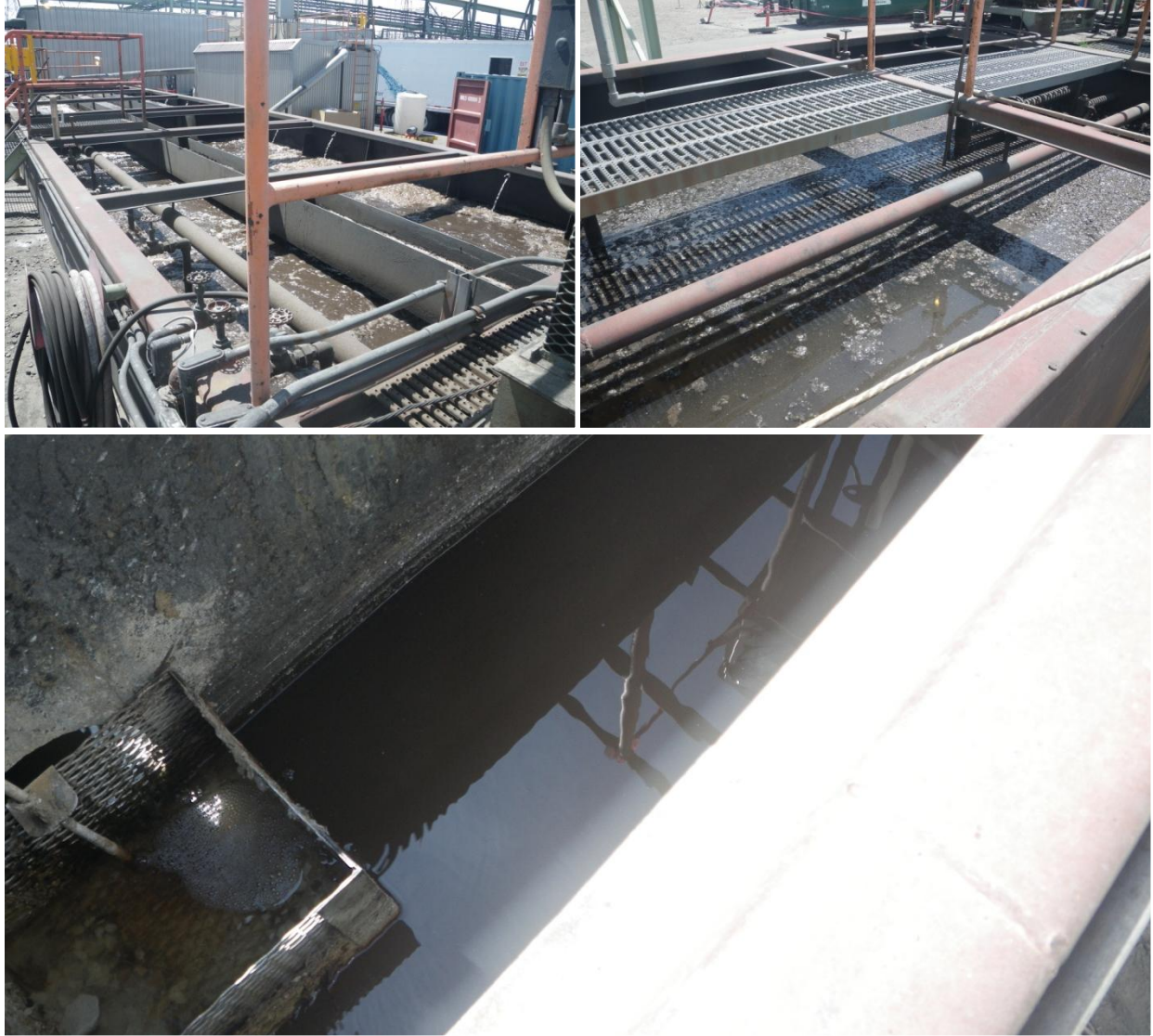
Figure 13: Domestic wastewater treatment package plant; final effluent (bottom) murky.
