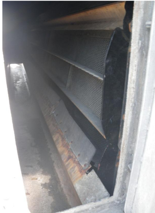
Figure 9: Cooling water intake channel and screens for units 4 and 5.
