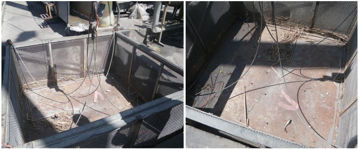
Figure 10: Fish return from traveling screens disposed of once/day. Approximately 12 fish between 1" and 6" observed in basket.
