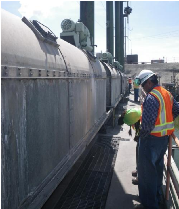
Figure 9: Cooling water intake channel and screens for units 4 and 5.
